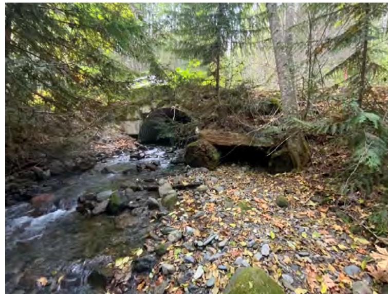
Looking at outlet from downstream.
