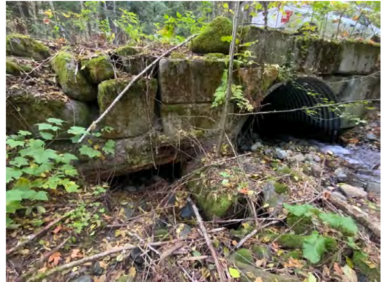
Inlet of both old log culvert and arch. Arch footing supported by log sill and old culvert supporting riprap
